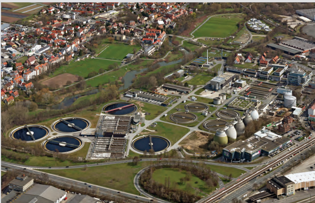
Sewage Treatment Plant No. 1 from the air. Photo: Nürnberg Luftbild, Hajo Dietz.
